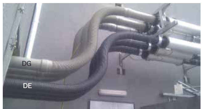
DG Type 12kV / 4000A and DE type 12kV / 3150A
