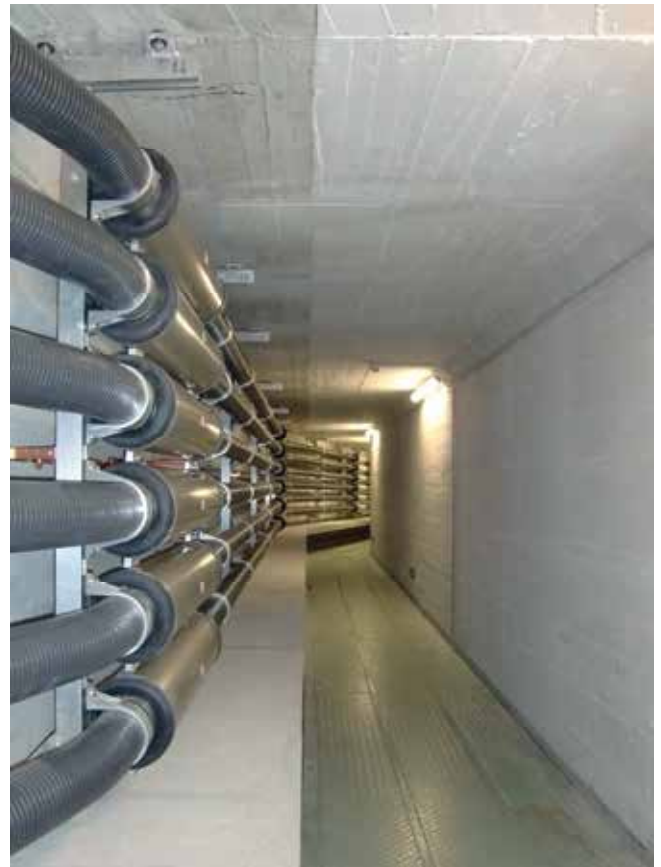
1350m of busbars have been installed
