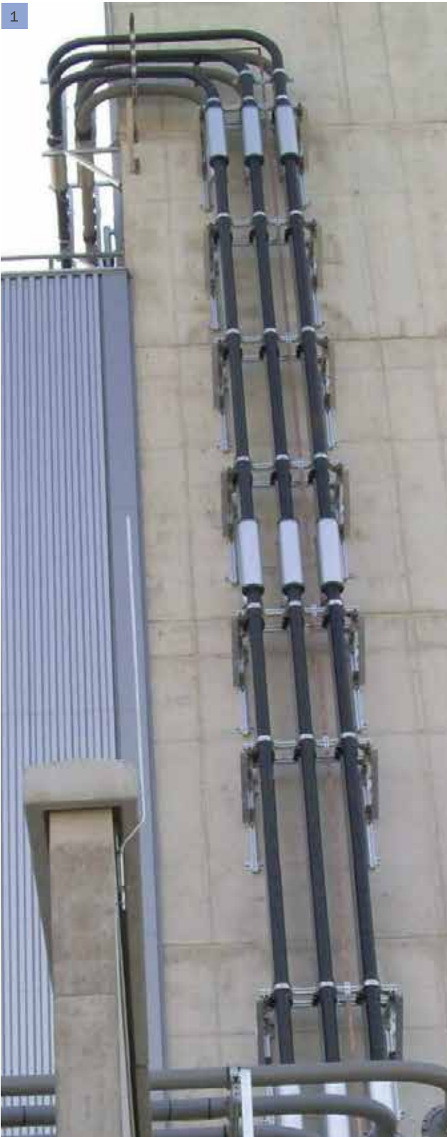
1 GuD Linz / Austria 25m long in vertical position No additional protection is needed for outdoor application.
