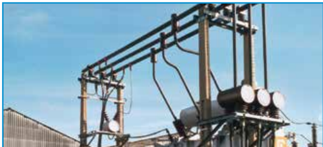
GASLINK® SF 6 insulatet busbar system
